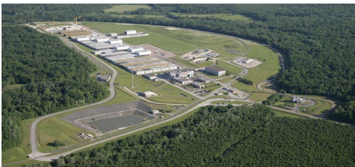
▲ The French low and intermediate level waste repository, in the Champagne region.
